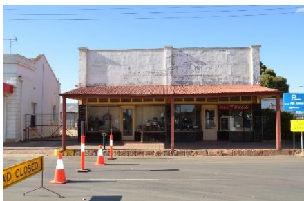
109-111 Main Street: Prior to commencement of the Main Street Project
